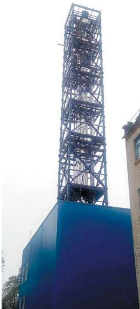
Fig. 3. Liquid effluent detritization plant commissioned by FSUE "RosRAO"
