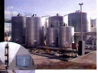
Module formaldehyde/UFC 85 plants with high degree of prefabrication located directly at woodwork plants are capable of satisfying needs of the plant in raw materials for production of adhesives in situ.
